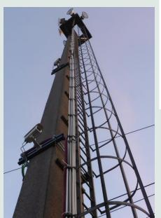
The system consists of two motion-triggered cameras. One is mounted at the height of the overhead line to inspect the wear of the pantograph. The second is mounted higher at approximately 10 m and looks for damage and defects. The second camera also enables vehicle identification.
